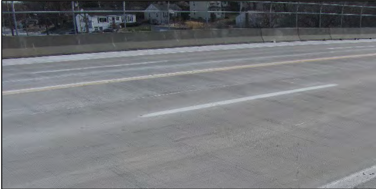
Figure 171. Typical RC bridge railing condition for Bridge Number 15558X.
