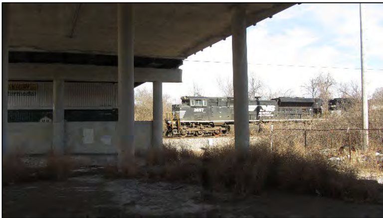
Figure 114. Freight train passing below Bridge Number 15558X
