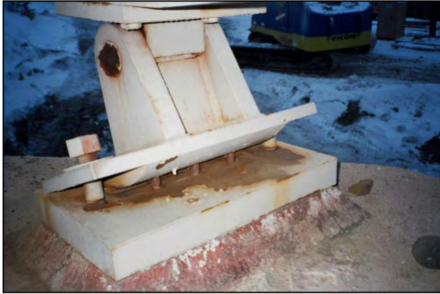
Figure 145. Misaligned rocker bearing. (Source: Alaska DOT)
