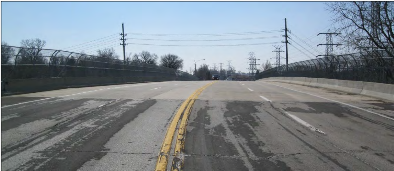
Figure 4. Approach view to Bridge Number 15558X, looking south.
