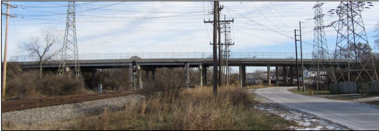
Figure 76. Elevation view of Bridge Number 15558X, looking east.
