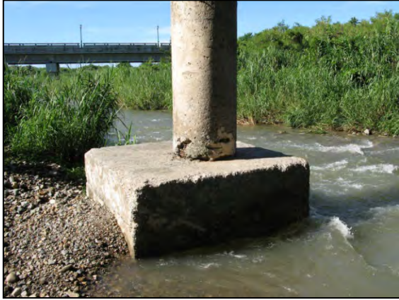
Figure 153. Exposed column footing in stream.
