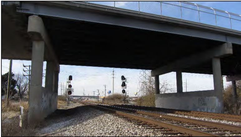
Figure 113. Bridge elevation view of two railroad tracks below Bridge Number 15558X.
