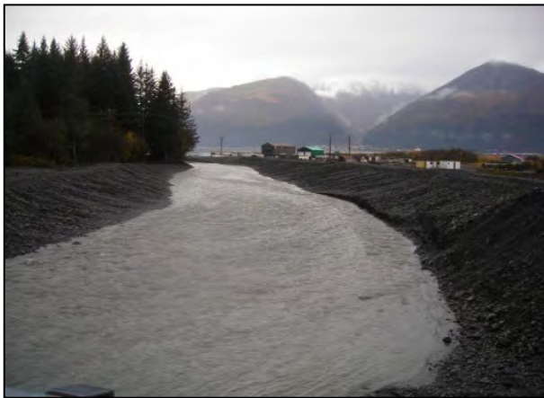
Figure 151. Looking downstream from bridge at excavated material. (Source: Alaska DOT)
