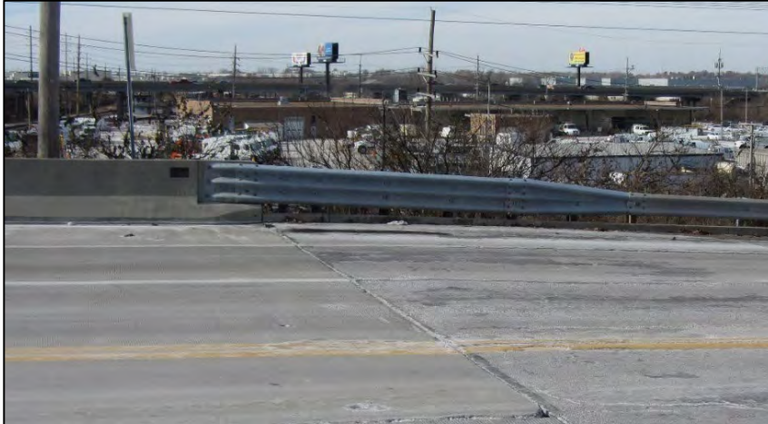
Figure 13. Reinforced concrete bridge railing and metal transition railing for Bridge Number 15558X.
