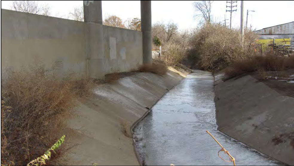
Figure 124. Berkeley Branch Coldwater Creek below Bridge Number 15558X.
