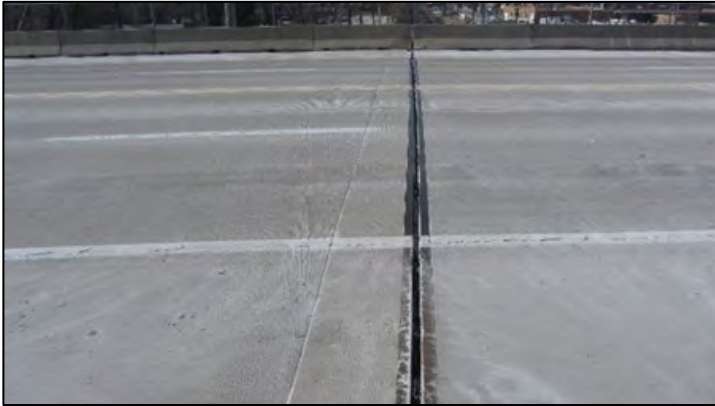
Figure 176. Strip seal bridge joint for Bridge Number 15558X.
