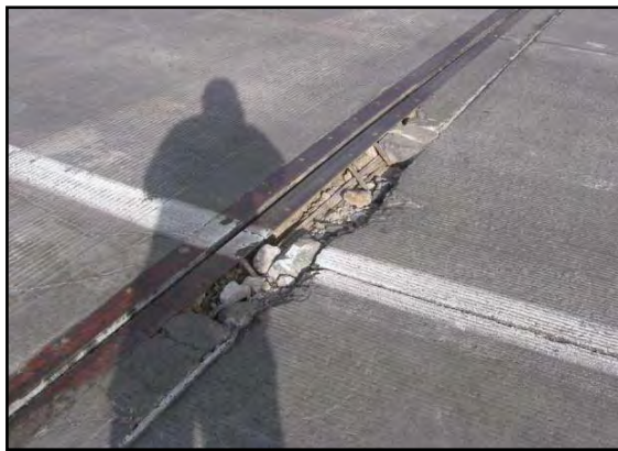
Figure 148. Spall in joint header. (Source: Colorado DOT)
