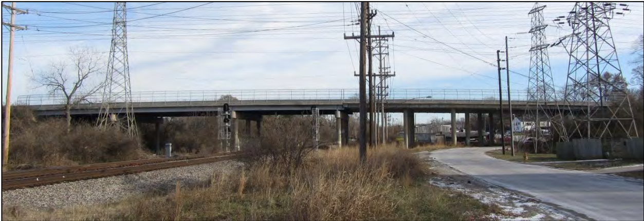
Figure 2. Elevation view of Bridge Number 15558X, looking east.
