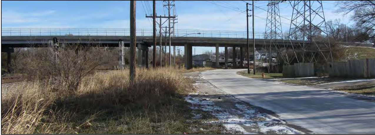
Figure 6. Elevation view of the North Hanley Road Bridge, looking east.
