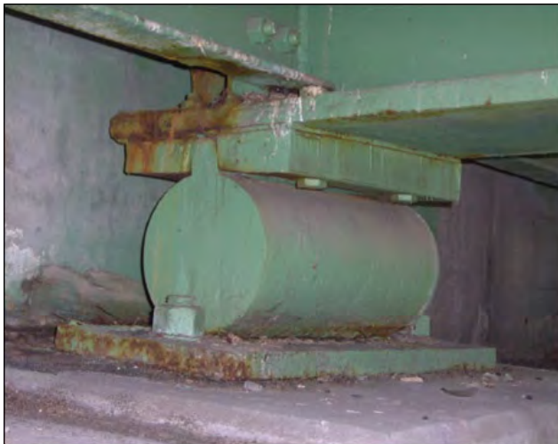
Figure 146. Surface rust on moveable bearing.
