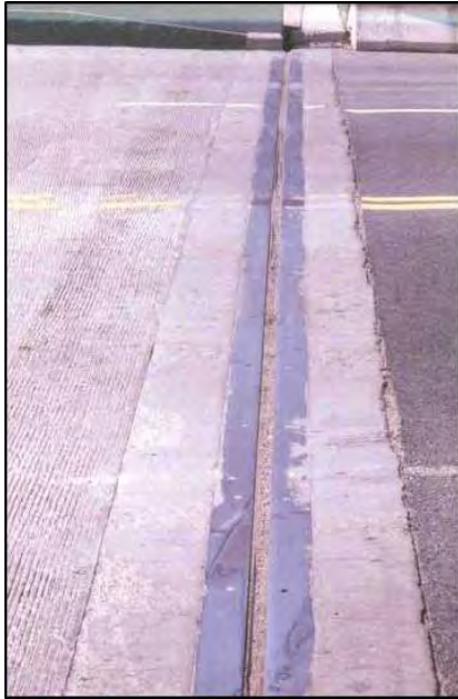
Figure 147. Joint partially filled with debris.
