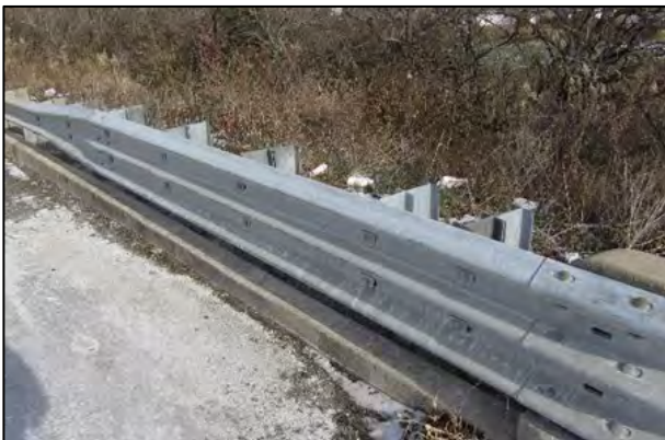
Figure 172. Typical condition of thrie-beam bridge transition railing for Bridge Number 15558X.
