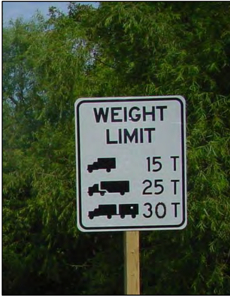
Figure 125. Approach view with load posting sign for Bridge Number 15558X.
