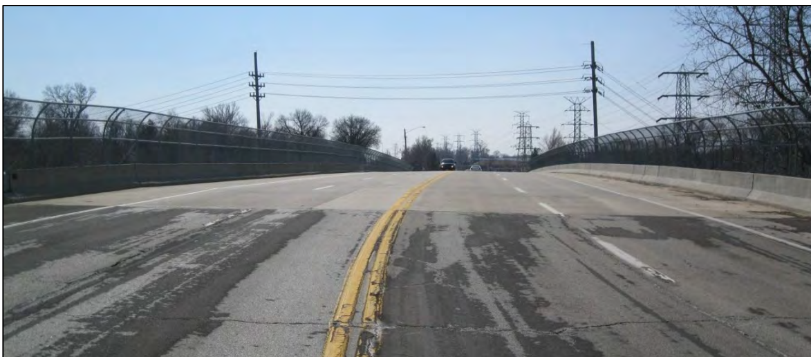
Figure 78. Approach view for Bridge Number 15558X, looking south.
