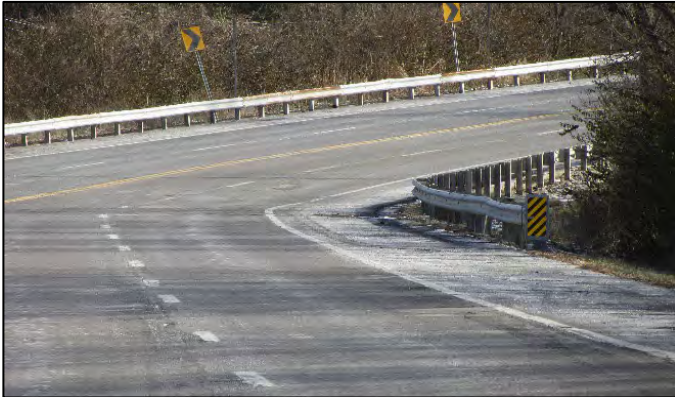
Figure 182. Approach roadway for Bridge Number 15558X, looking south.
